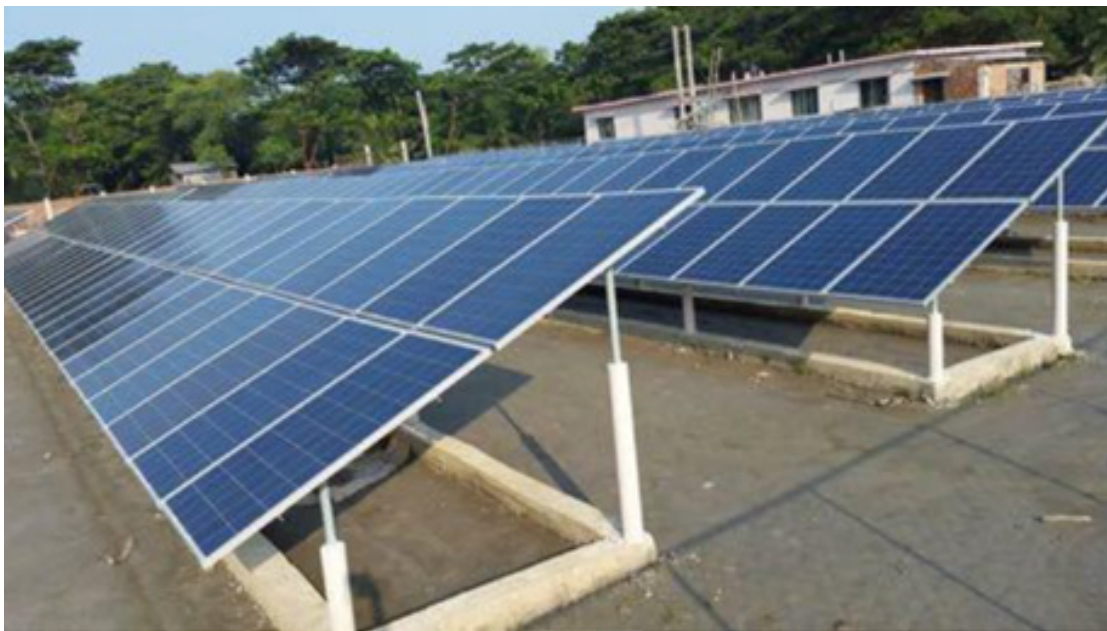
beam type foundation
